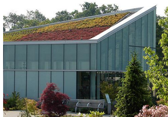
Figure 4.17 Green roof on Toronto Botanical Garden
