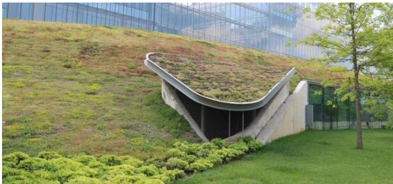
Figure 3.54 Round green roof on a hill
