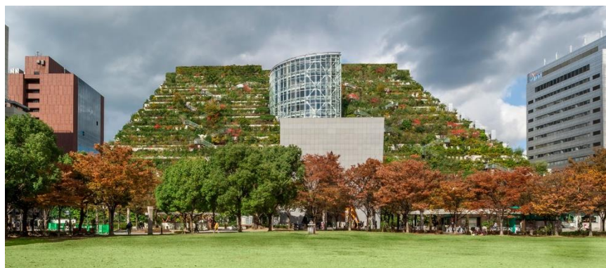
Figure 3.14 Intensive green roof on Acros Fukuoka Prefectural International Hall in Japan ( https://www.greenroofs.com/projects/acros-fukuoka-prefectural-international-hall/ ) [Accessed: 12.05.2021]
