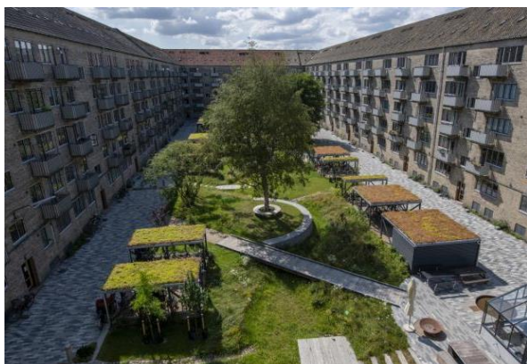
Figure 4.25 Green Roof on open-sided huts ( https://www.kk.dk/nyheder/nu-indvies-fremtidens-gaardhave-i-askoegade ) [Accessed: 28.12.2020]
