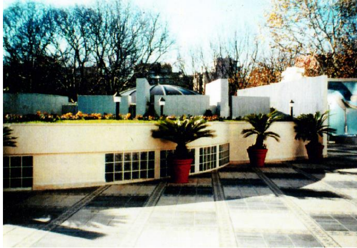
Figure 5.3 Green roof on Ceylan International Hotel (Köylü, 1997)
