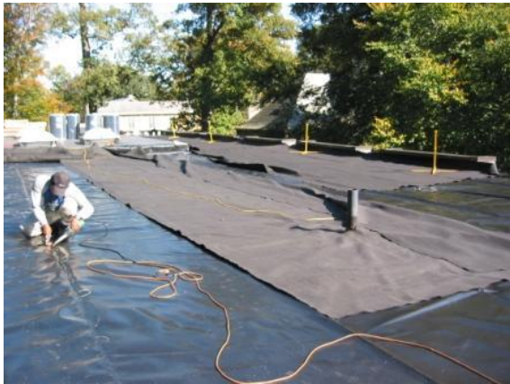
Figure 3.24 Root barrier
