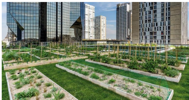
Figure 3.40 Planting beds on green roof ( https://zinco-greenroof.com/press-release/le-cordon-bleu-paris ) [Accessed: 10.12.2020]
