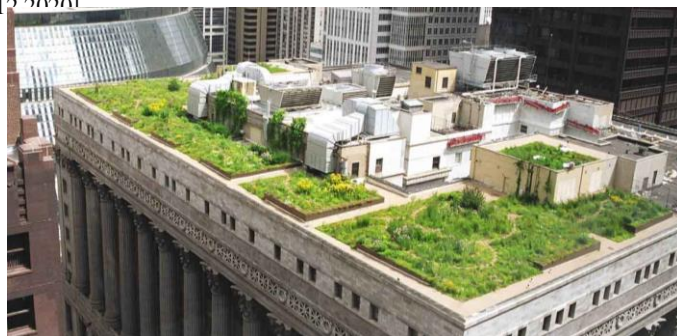
Figure 3.43 Green roof in Chicago City Hall
