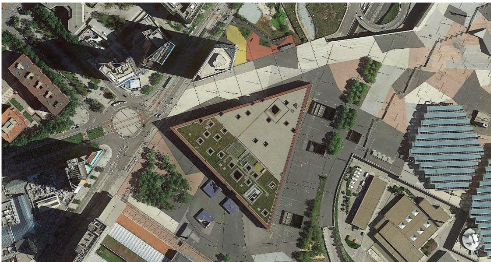
Figure 4.8 Aerial view of green roof on Natural History Museum
