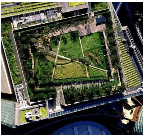
Figure 3.33 Roppongi Hills Rooftop Farm
