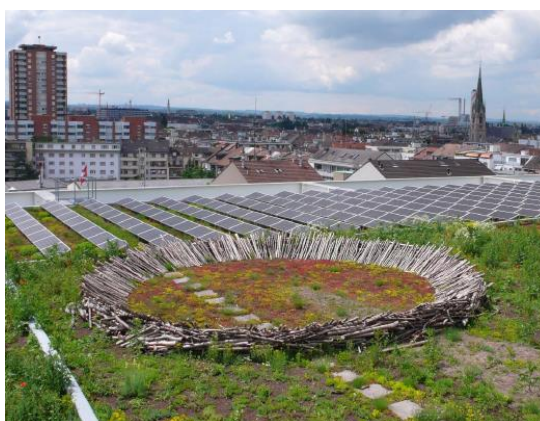
Figure 3.29 Green roof on Main Exhibition Hall in Basel
