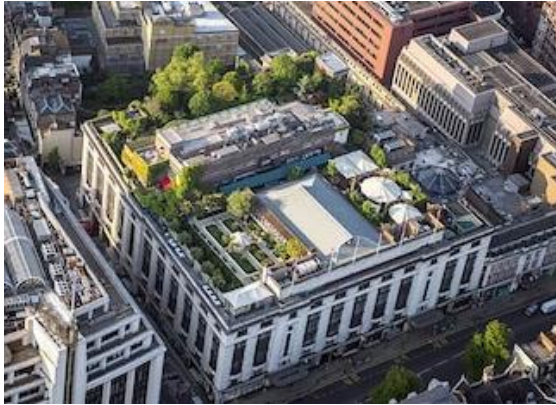
Figure 3.11 Top View of roof garden on Derry and Toms Department Store
