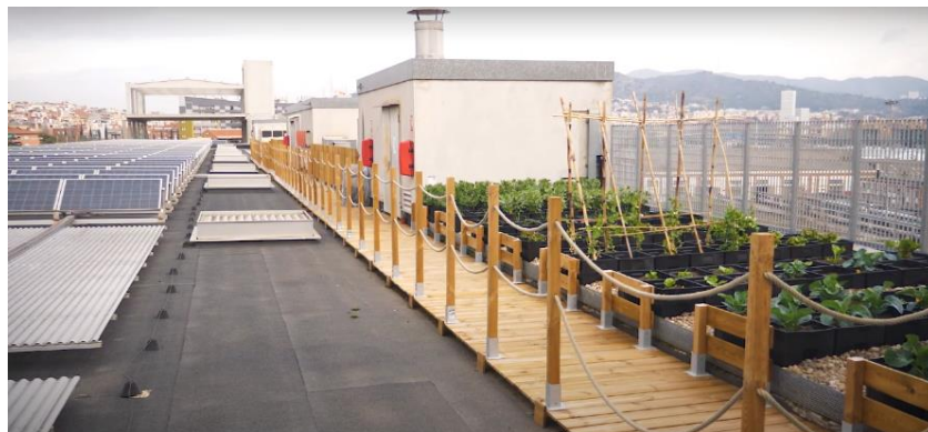
Figure 4.7 Cultivation spaces and solar panels on the green roof of TEB building ( https://ajuntament.barcelona.cat/ecologiaurbana/sites/default/files/noind/10propostesguanyadorecobertes.pdf ) [Accessed: 28.12.2020]
