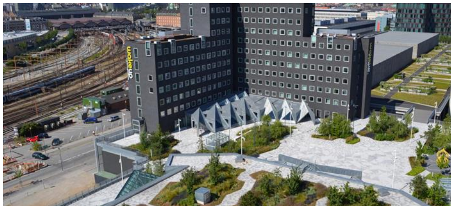
Figure 4.24 Green roof on Danish State Archives ( http://wsud-denmark.com/copenhagen-green-roof-the-danish-state-archives/home-page/34758 ) [Accessed: 28.12.2020]
