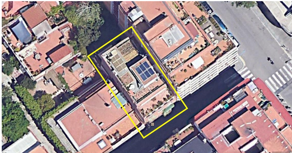
Figure 4.4 Aerial View of Green Roof in the street of Balcell
