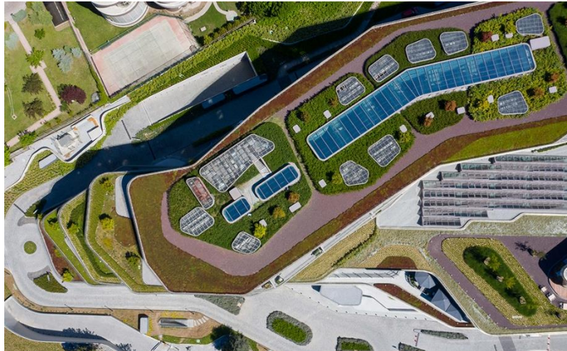
Figure 5.15 Top View of Green Roof on Kuzu Effect
