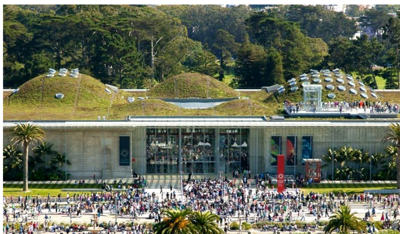
Figure 3.16 Semi-intensive green roof on California Academy of Sciences
