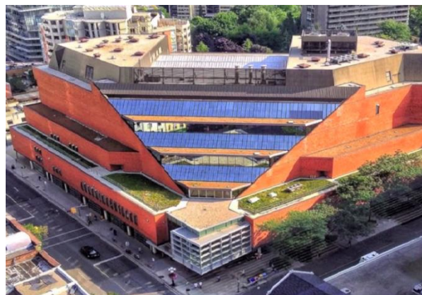
Figure 4.19 Aerial view of the green roof on the Gladstone Library
