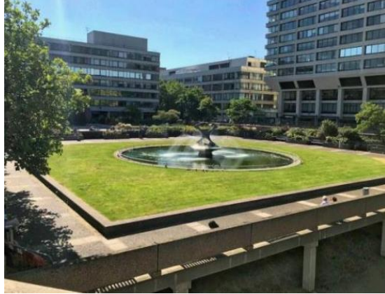
Figure 4.29 Green roof on St Thomas's Hospital
