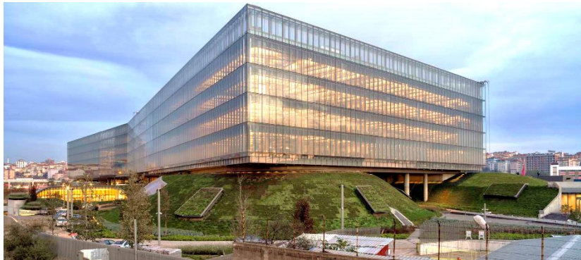
Figure 3.53 Green roof on Garanti Bank Technology Campus
