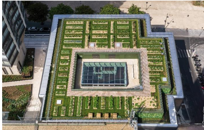
Figure 3.39 Top view of Le Cordon Bleu ( https://zinco-greenroof.com/press-release/le-cordon-bleu-paris ) [Accessed: 10.12.2020]
