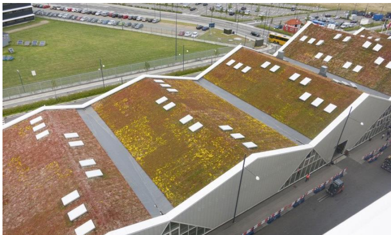
Figure 3.18 Extensive green roof on Copenhagen cruise ship terminal
