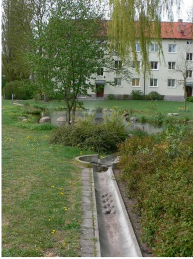
Figure 2.4 Stormwater canal at the Eco City Augustenborg
