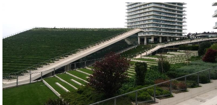
Figure 5.10 Extensive Green Roof on Performing Arts Center (Personal Archive)
