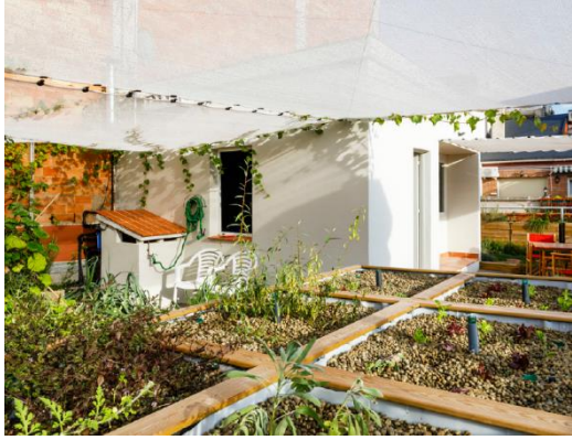
Figure 4.2 Green roof in the street of Balcells
