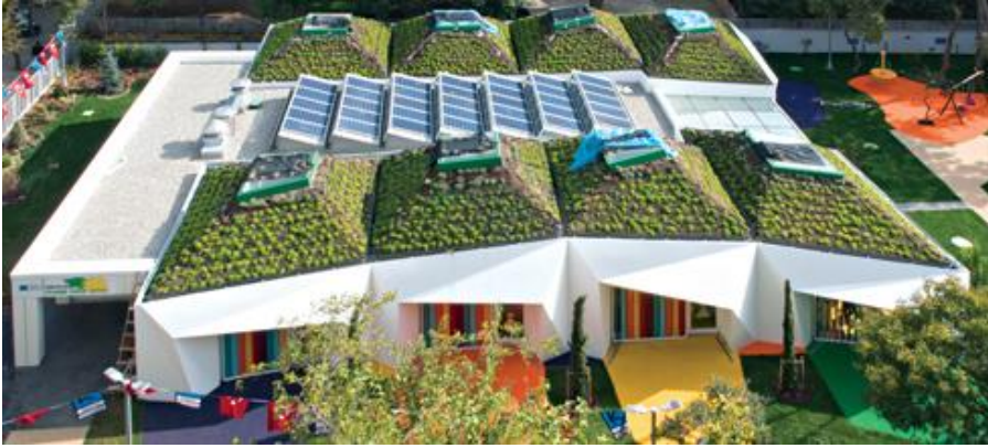
Figure 5.12 Green roof on Bahriye Üçok Kindergarten
